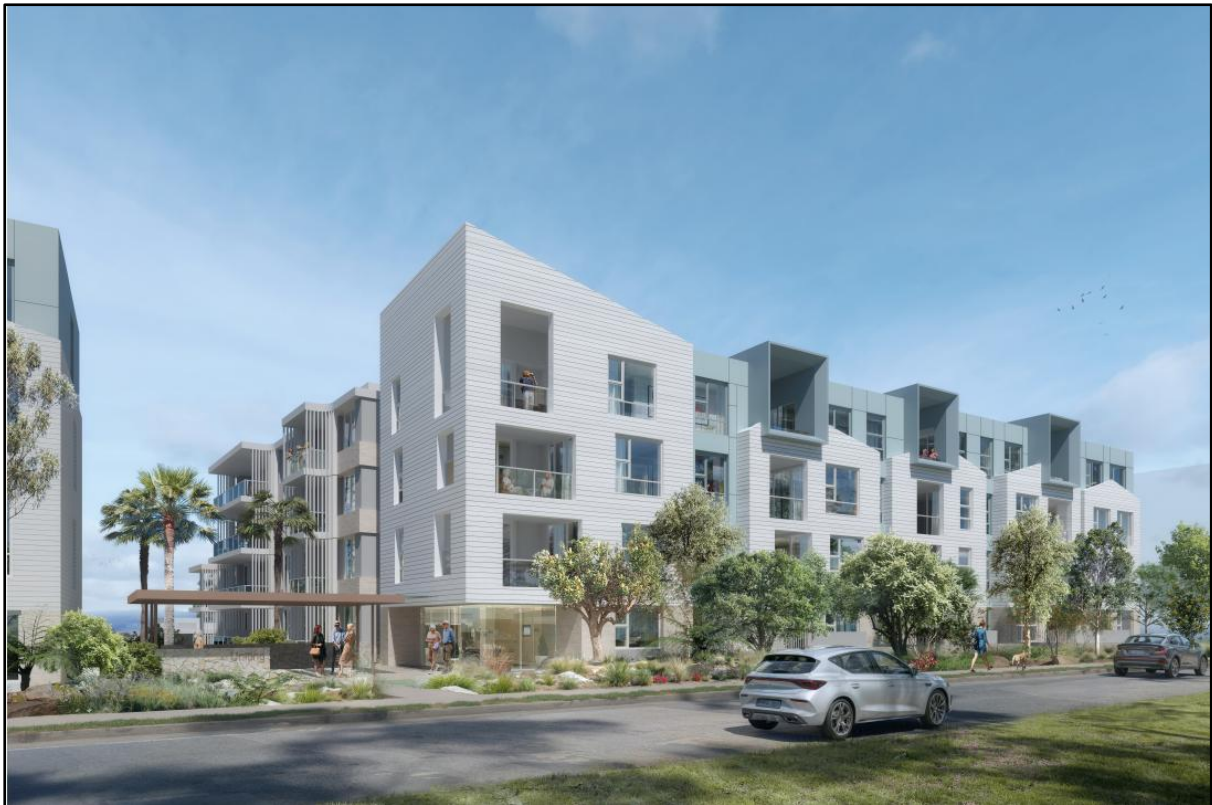
Figure 6: Building R3 along Wattle Road
